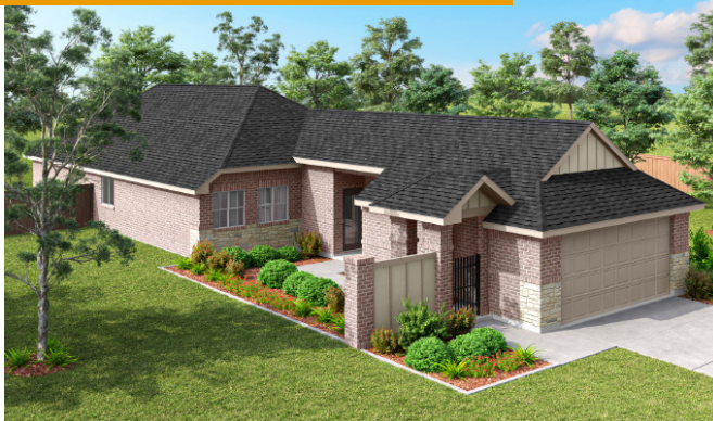
ELEVATION A - Brick Wing Wall
