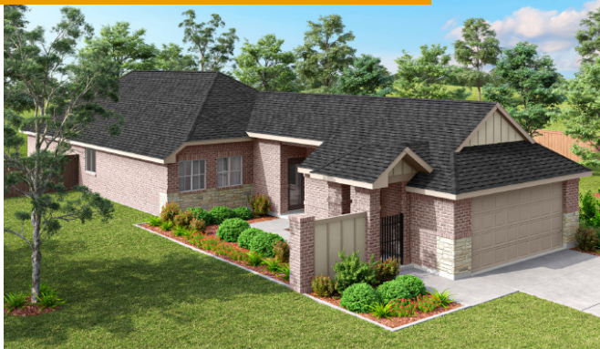
ELEVATION A - Brick Wing Wall
